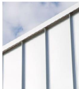
METAL STANDING SEAM CLADDING
